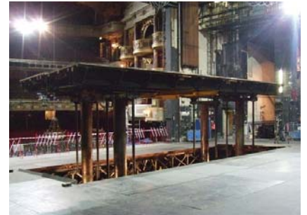
Drury Lane Theatre's hydraulic stage bridges.
