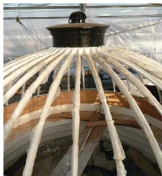
Fixing the dome of the roof light at St Martin-in-the-Fields School.
